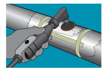
4. Using the Transmitter unit as a guide, roughly indicate the area to be cleaned using masking tape (see above).
